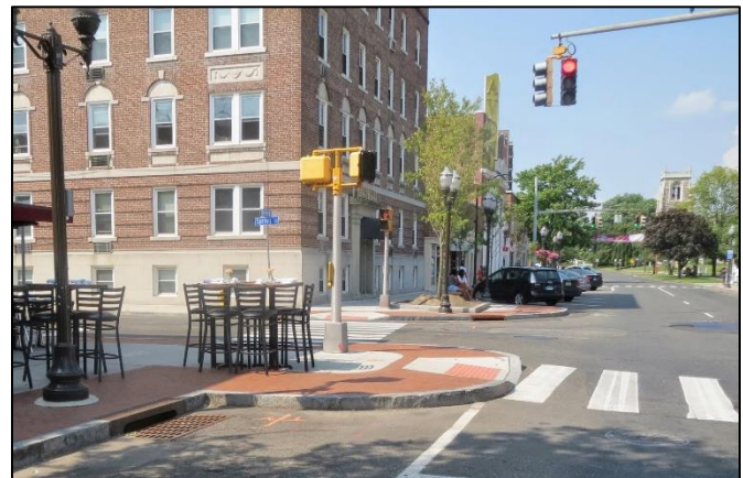
Example of a curb bulb-out at a signalized intersection.
